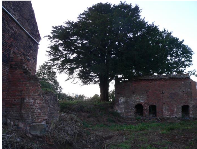
Yew Tree in North West Corner.
